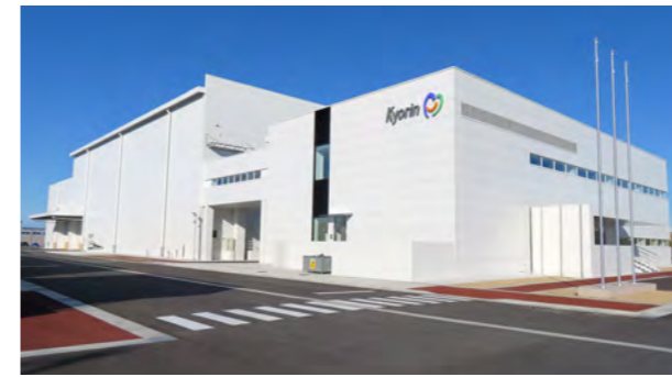
Takaoka Plant Location: Takaoka, Toyama
