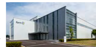
Takaoka Pharmaceutical Technology Innovation Center
